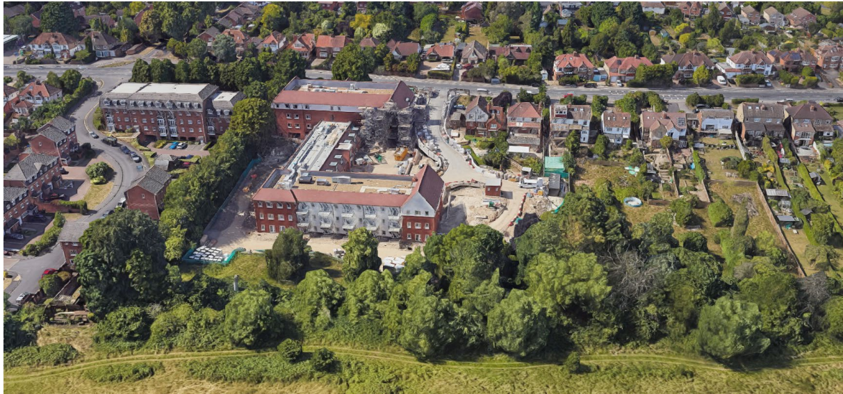
Figure 3: Aerial view looking north (Signature care home to the west under construction at this time)
